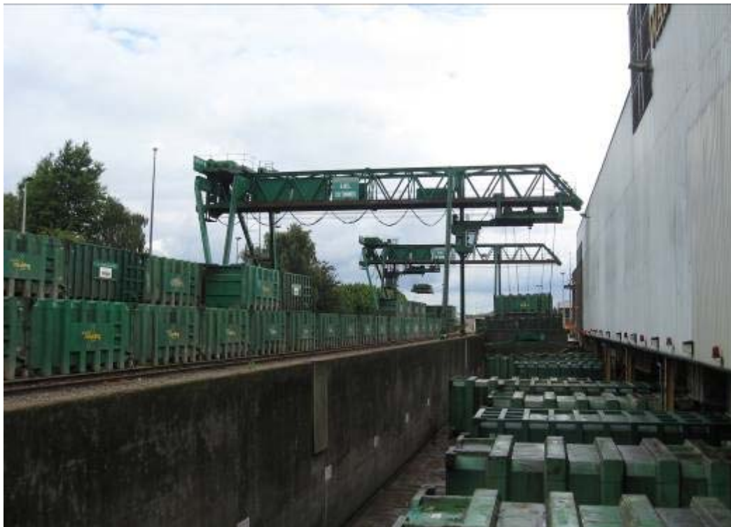
Waste container loading bay at the rail handling facility at Hendon
